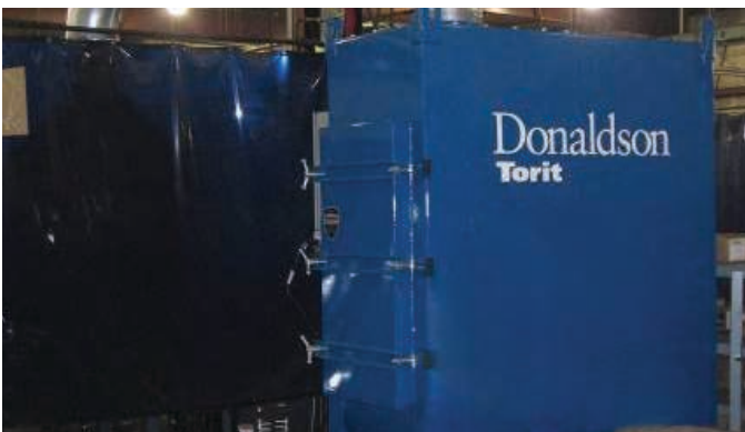
TG4 on Welding
